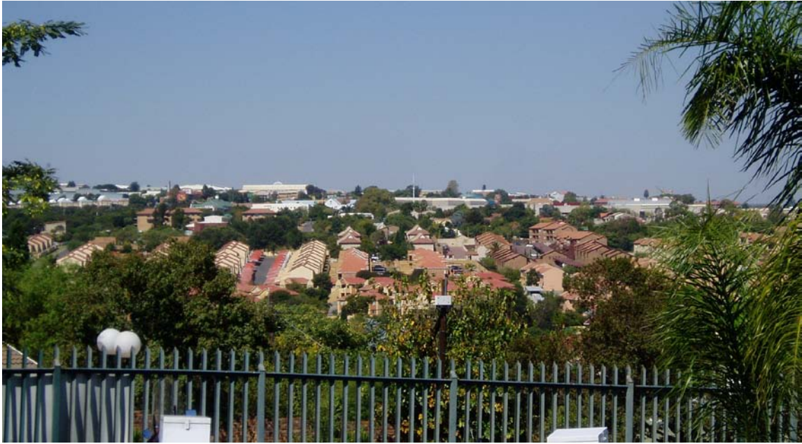
Town house development
